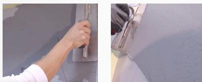
Remove the protective tape before the Microcement hardens and allow the second layer Microcement Base.
