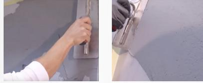
Remove the protective tape before the Microcement hardens and allow the complete drying of the second layer of Microcement Base AQUA.
