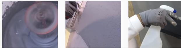
The union between the first and second layer will give a final thickness of 1,5 mm approximately.
